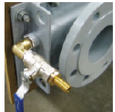
Drain valve QLKZ-04-21.
